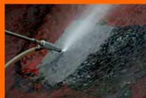
Surface – Sand Blasting
