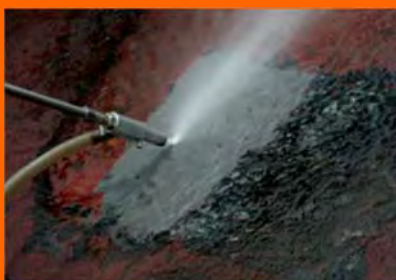
Surface – Sand blasting
